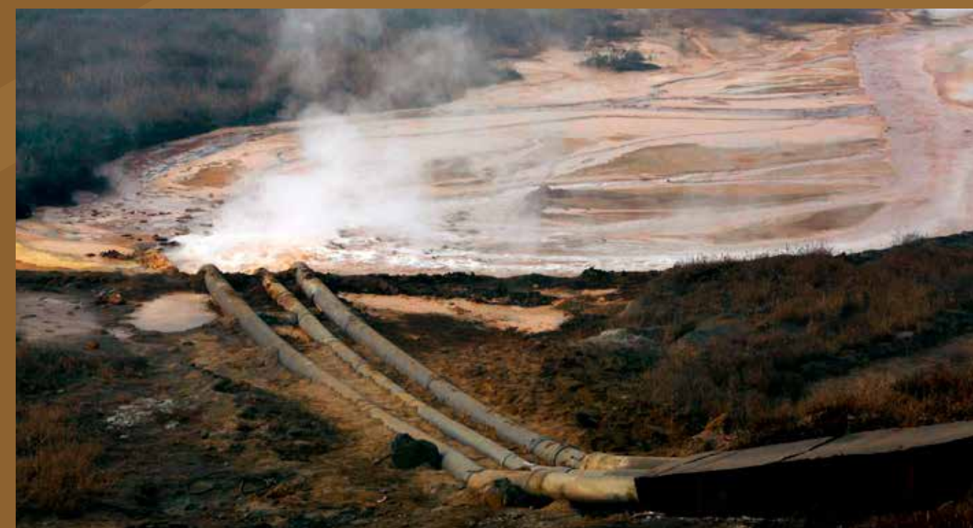
Figure 24: Image of tailings pond at Bayan Obo .
