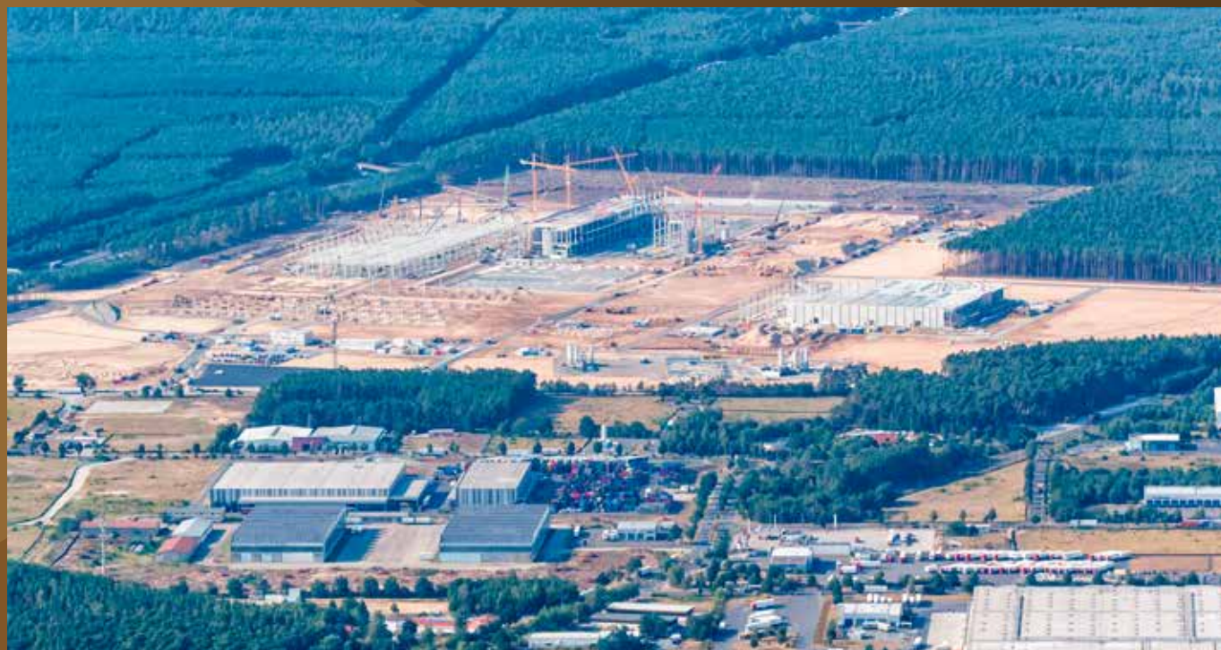
Figure 72: Tesla's new Berlin Brandenburg Gigafactory Under Construction In Berlin
