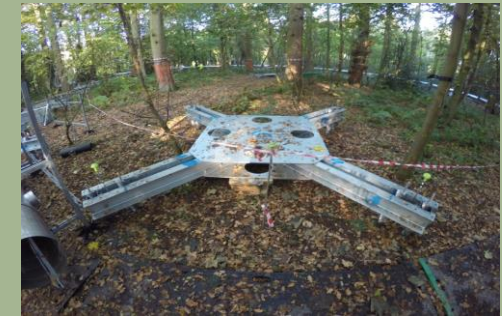
Fig 1. Typical FACE Array Grillage with piles installed
