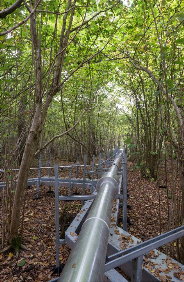
Figure 5 Some of the 1000m of pipework running through the forest
