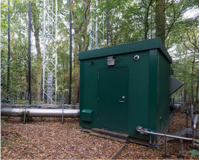
Figure 7 The FACE control sheds
