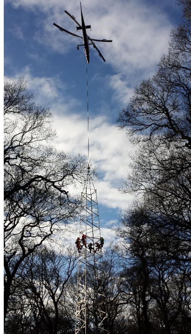
Figure 8 Installing the large flux tower using a helicopter
