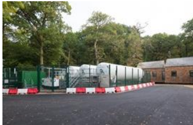
Figure 2 Access road, CO 2 tankers and welfare units
