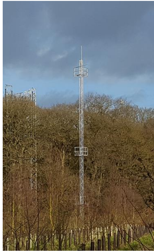
Figure 5 The South west met mast, one of four erected in 2017 to measure air flow into, out of and over, the forest
