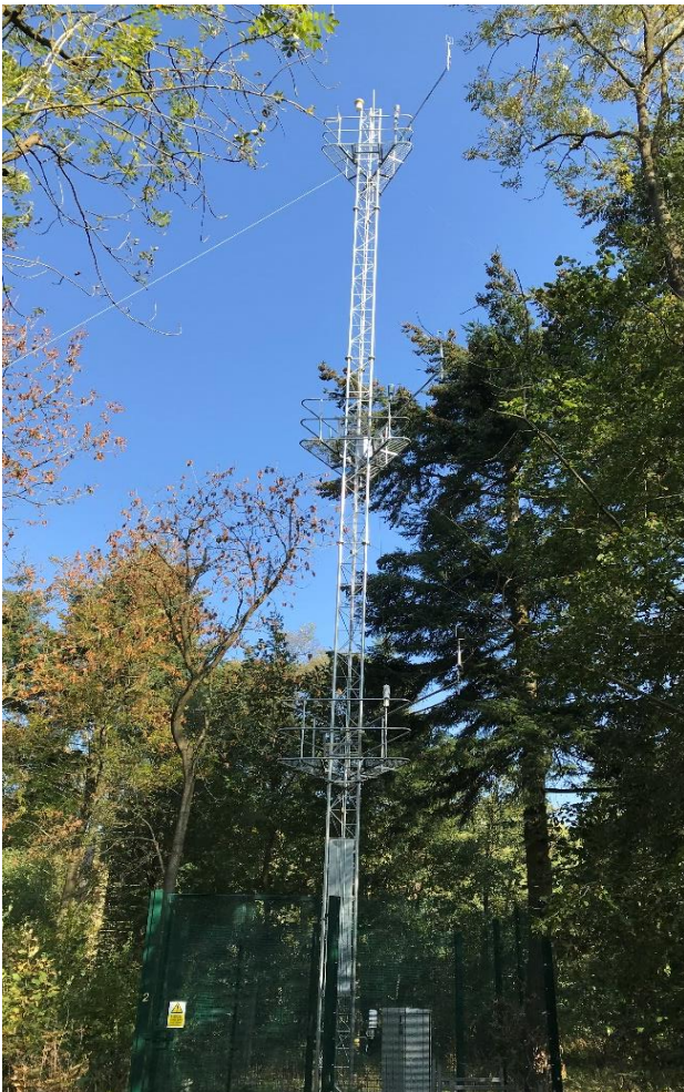
One of four instrumented met masts to measure air flow into, out of and over, the forest
