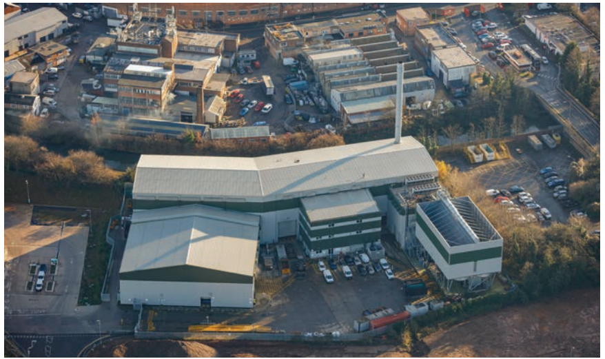
FIGURE 28: TYSELEY ENERGY PARK WOOD GASIFIER (ABOVE) AND LOW-CARBON FUEL STATION (BELOW). SOURCE: WEBSTER AND HORSFALL
