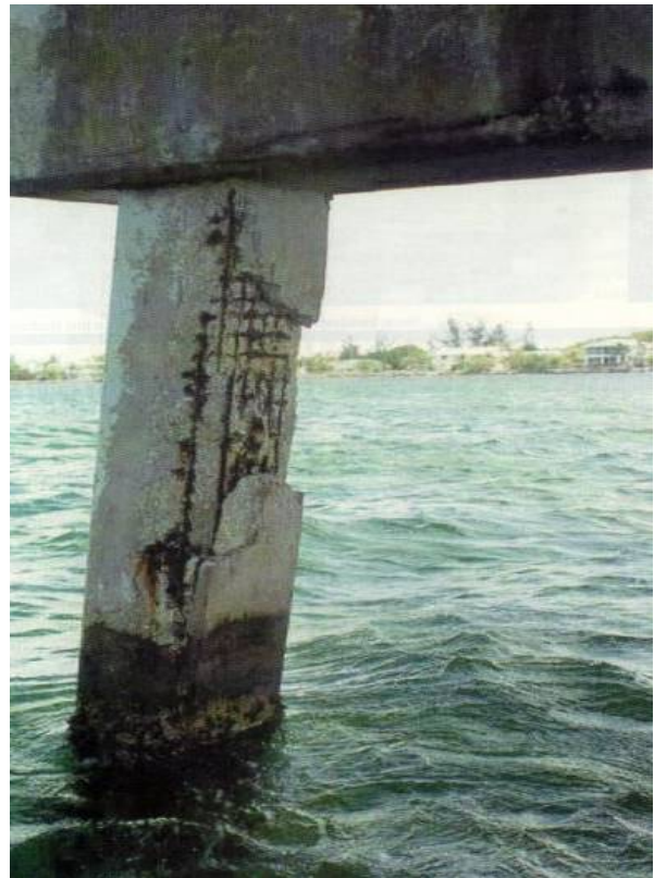
Figure 2: Spalling of concrete cover due to corrosion of reinforcing steel.
