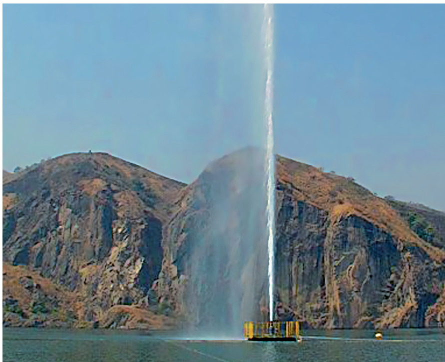
Engineers venting carbon dioxide from Lake Nyos to prevent a repeat of the 1986 disaster
