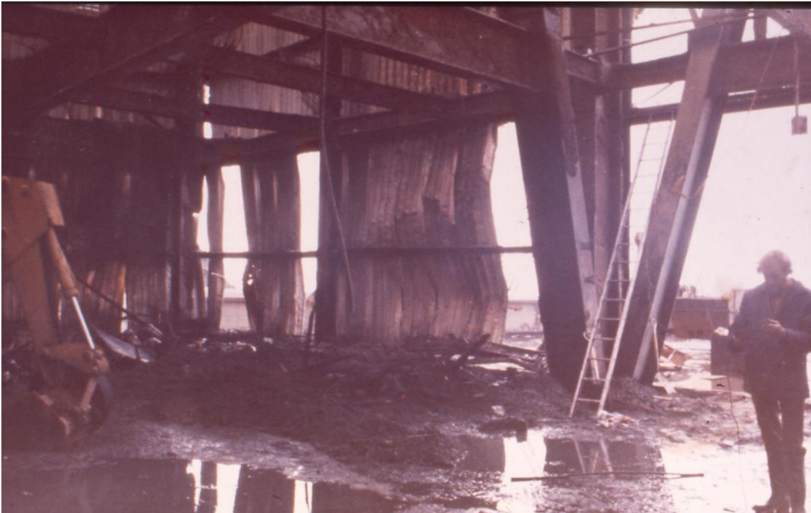
Figure 6.6: The remains of the inner face of the Galbestos wall. A wall of combustible Decalin fibreboard had been erected inside Summerland parallel to the Galbestos wall creating a 12 inch concealed void.
