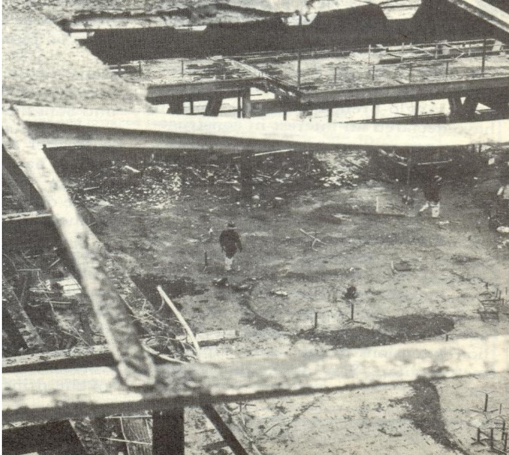
Figure 6.14: Scene of complete devastation: the Solarium viewed through the Oroglas roof after the fire. Note how the metal table legs survived the fire. The main entrance is near the top right-hand corner of the photograph.
