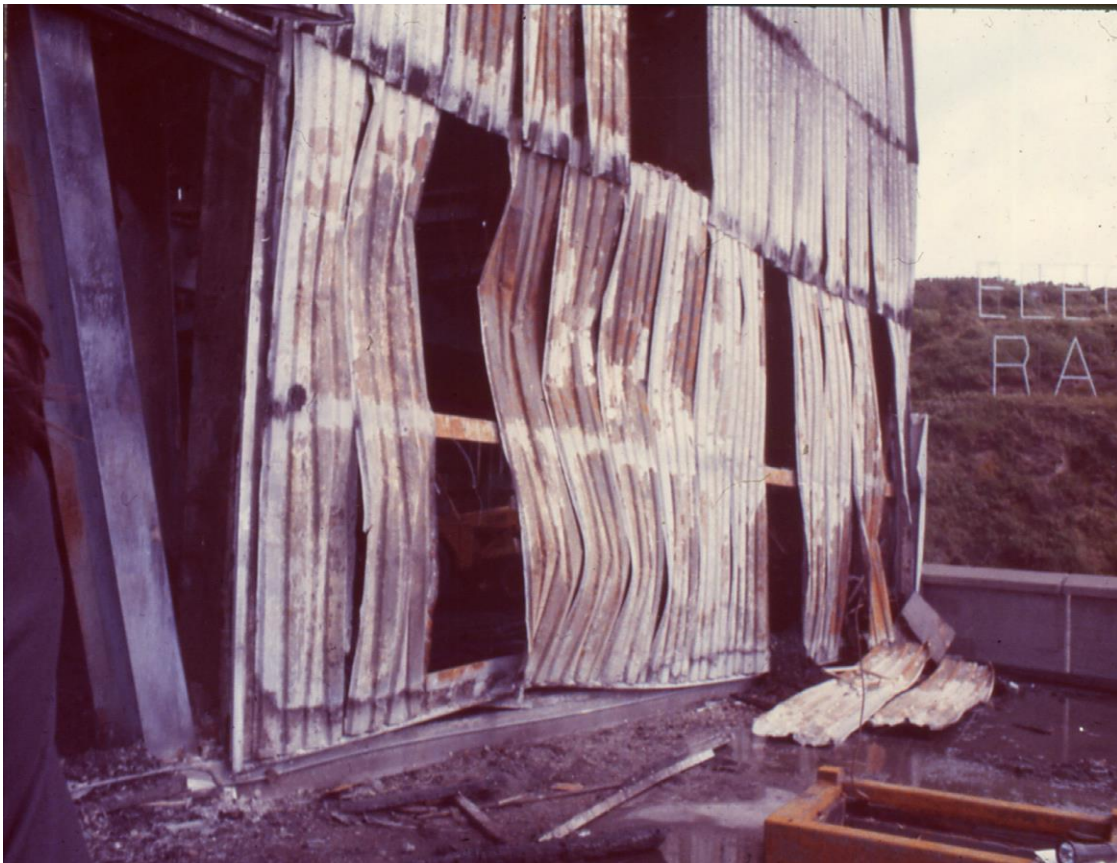
Figure 6.3: The deformed Galbestos wall after the fire (Photograph: John Webb; Copyright Fire Research Station (FRS) and Building Research Establishment (BRE)) (This photograph appears with the written permission of BRE Global.)
