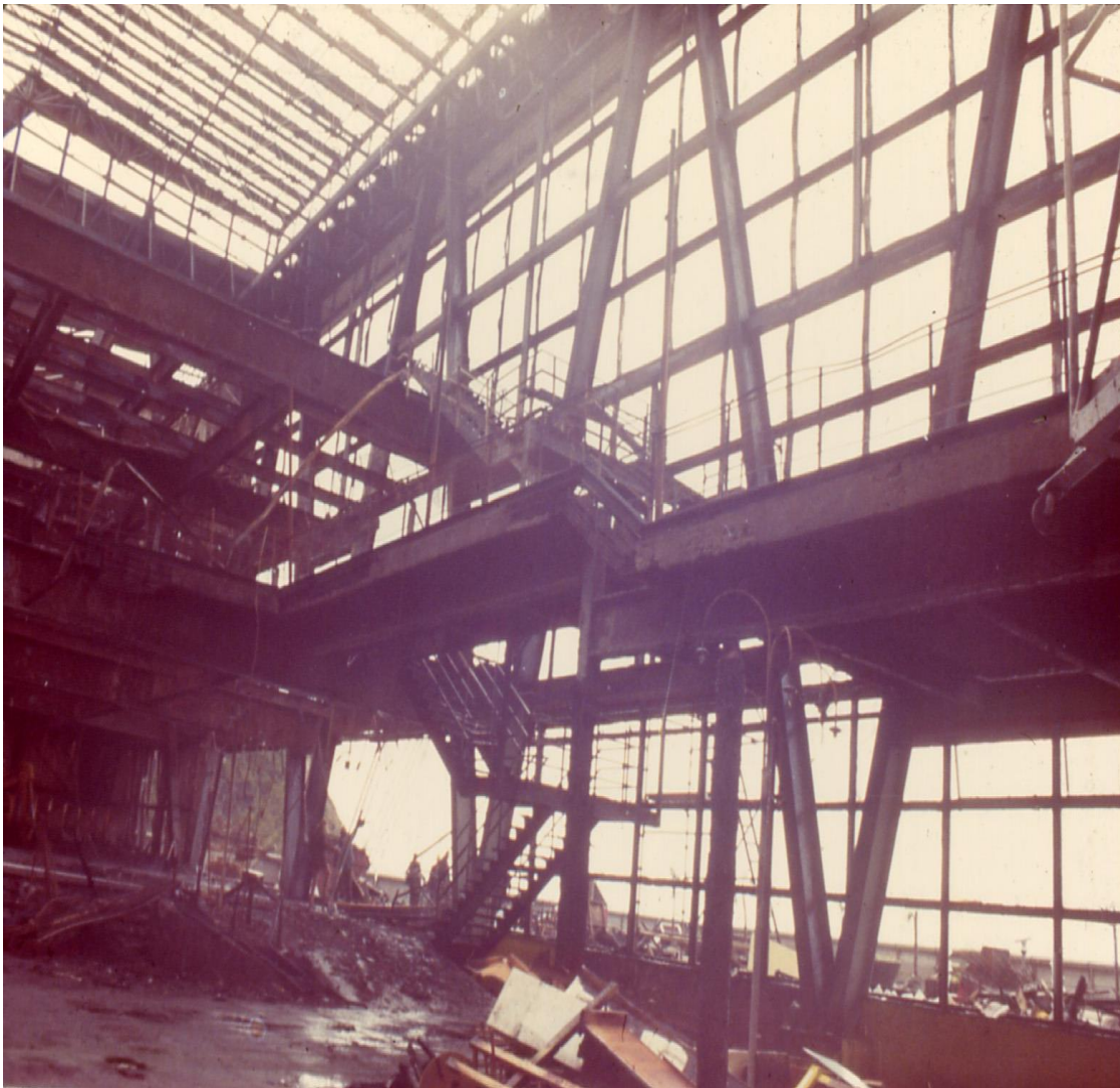
Figure 6.23: The Flying Staircase “created a wholly unnecessary hazard” (Photograph: John Webb; Copyright FRS/BRE). This photograph appears with the written permission of BRE Global.
