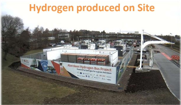
Hydrogen is produced for the first Aberdeen (bus) refueller at Kittybrewster by electrolysis of water.
