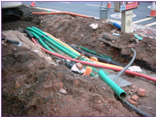
Crowded and haphazard use of near surface underground space in urban environments
