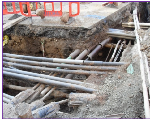
Crowded and haphazard use of near surface underground space in urban environments
