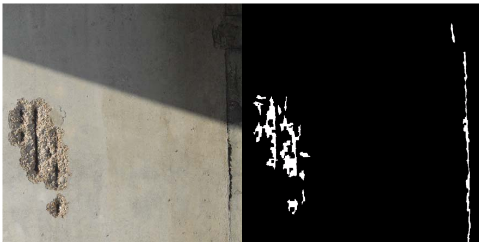
Figure 2: Example of segmentation of a defect from image (left) to segmented image (right).
