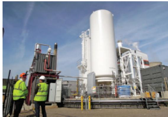
Figure 4: Highview's Liquid Air Energy Storage demonstration plant at Slough. The tank holds 60 tonnes of liquid air. Photo: Highview Power Storage
