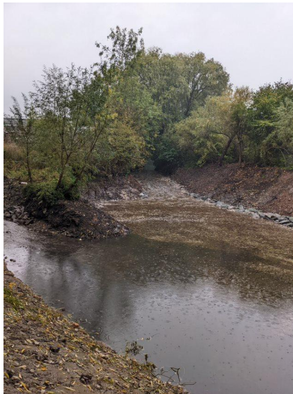
Ackers Weir - After Removal
