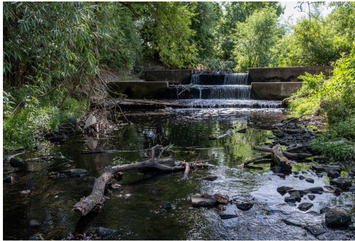
Ackers Weir - Before Removal
