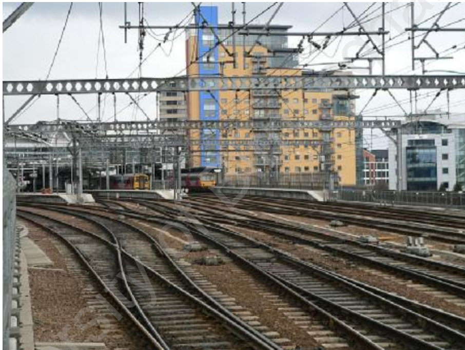
Figure 6 – Leeds station approach, OLE gantries and wiring in evidence (Chris McKenna)
