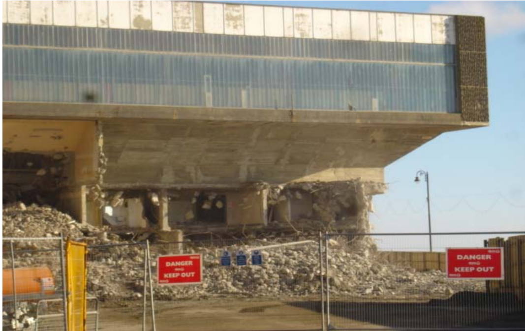
Figure 7.3: The demolition of the Aquadrome
