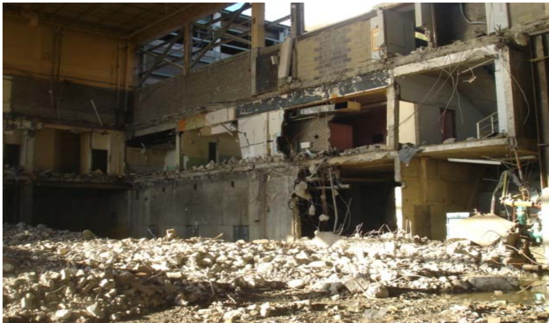
Figure 9.4: The demolition of Summerland. This photograph was taken in the Sports Hall. The remains of the Carousel staircase that descends from the Piazza floor to the Derby Bar can be seen on the right-hand side of the photograph (Photographs: Ricky Rooney and James Turpin)
