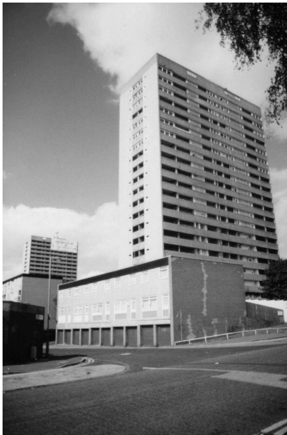
Figure 4: 22-storey tower blocks in the Cregoe Street area of Lee Bank, just prior to demolition. (Author, September 2000)
