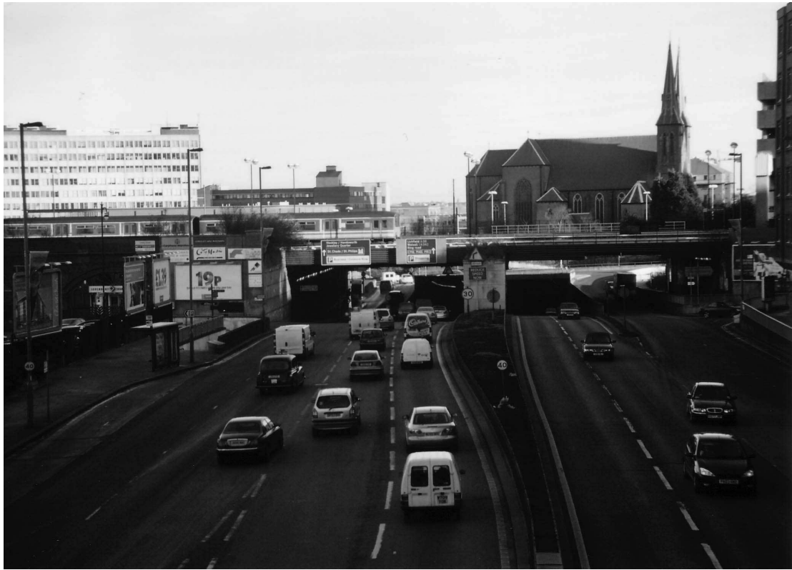
Figure 1: Western section of Birmingham's inner ring road. Built in a series of tunnels this portion of the road continues to operate in its original 1960s configuration (Author, January 2005)
