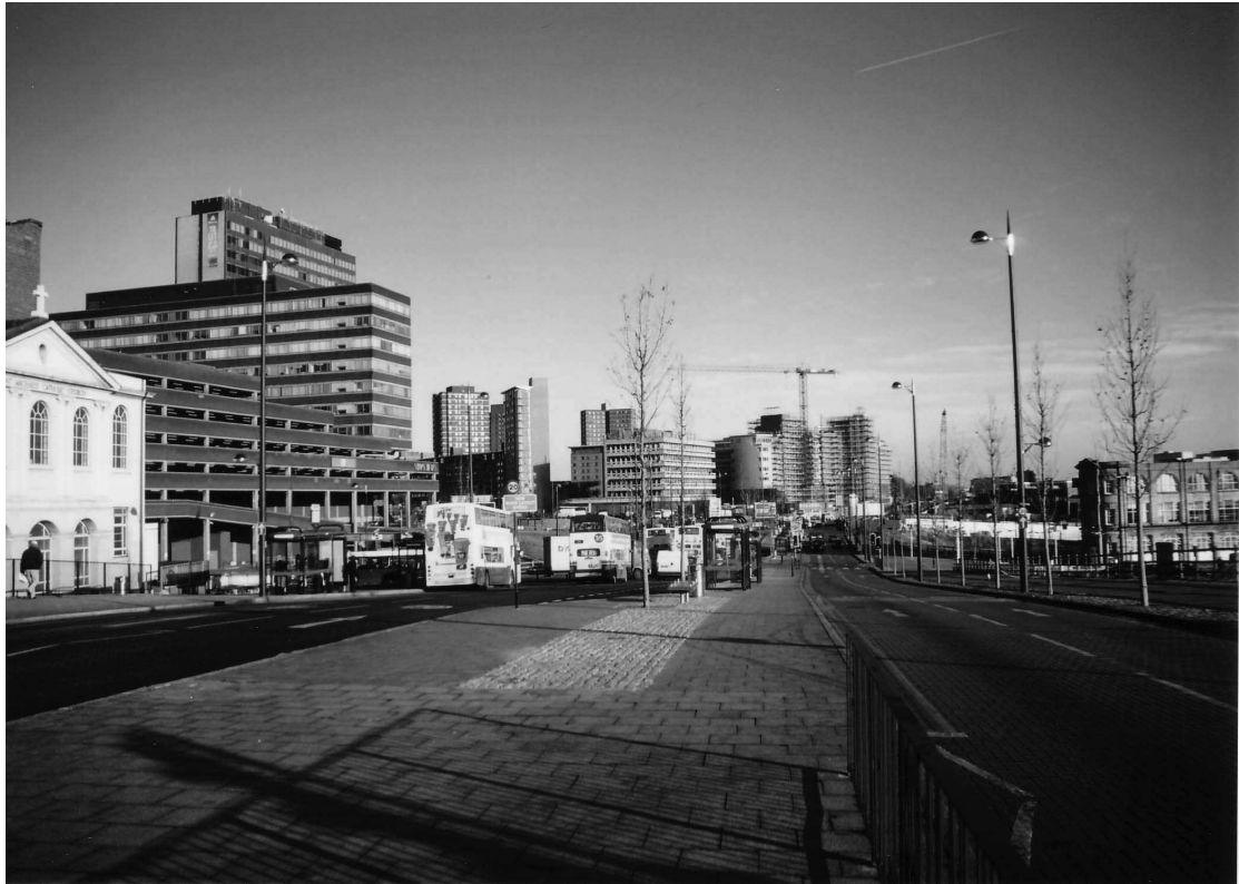
Figure 5: This boulevard replaces a very large multi-level interchange (Masshouse Circus) which was demolished in 2002 as part of the changes to the inner ring road on the eastern side of the city. (Author, January 2005)
