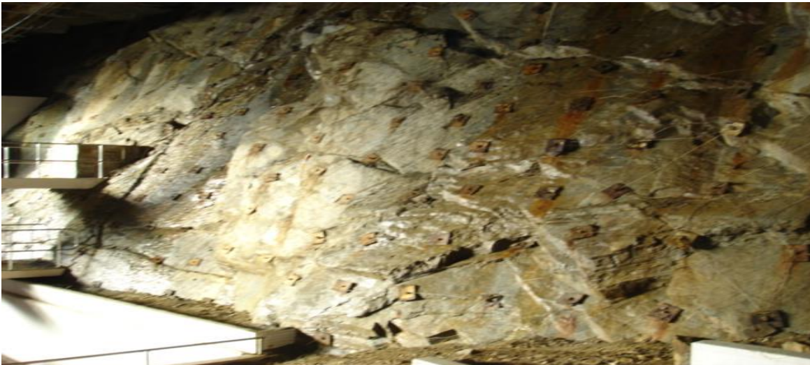
Figure 2.6: The cliff face formed the Aquadrome's fourth wall. Note the extensive bolting required to stabilise the cliff face (Photograph: Ricky Rooney and James Turpin)
