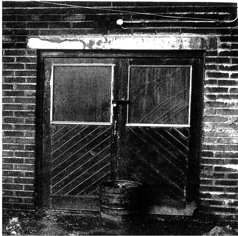
Figure 5.5: An exit door presumably at the eastern end of the building padlocked and obstructed by a beer barrel
