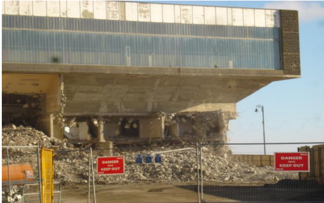
Figure 7.3: The demolition of the Aquadrome
