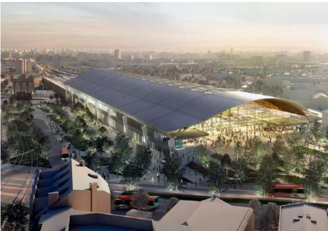
A new vision of the future Curzon Street Station. The original cellular glass roof has been replaced with a cheaper alternative (source: HS2)
