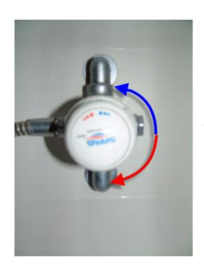
To increase the temperature turn the main body of the shower unit, the further you turn the control the hotter the water temperature. As a guide the control indicates settings from 1-9 if you feel the temperature is too hot or only warm at level 9 then please contact reception and ask to have the temperature checked and adjusted if necessary.
