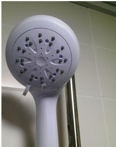
Where fitted the outer ring of the shower head (illustrated above) can be rotated to provide different settings for the jets of water, from a full wide spray to a small firmer jet
