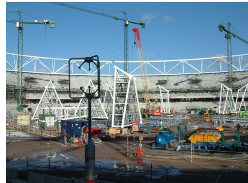
Testing at the Olympic park construction site
