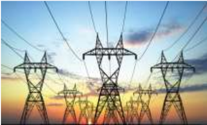
Smart Electricity and Gas Networks
