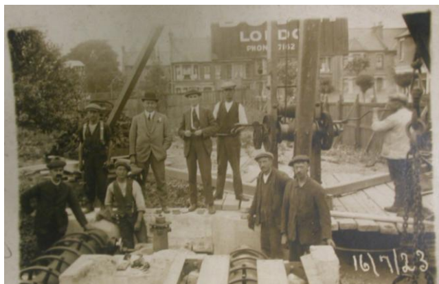
W. Y. Lewis and workforce, Southend demonstration site, 1923
