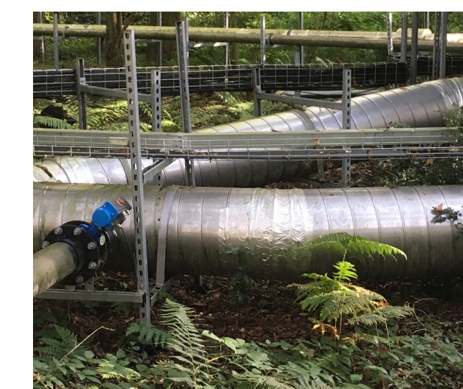
Pipes transporting CO 2 air mixture, elevated from forest floor
