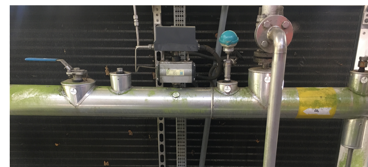
Pipes connecting carbon dioxide evaporators, super heater and decompressors. Flow controlled via pneumatic actuators
