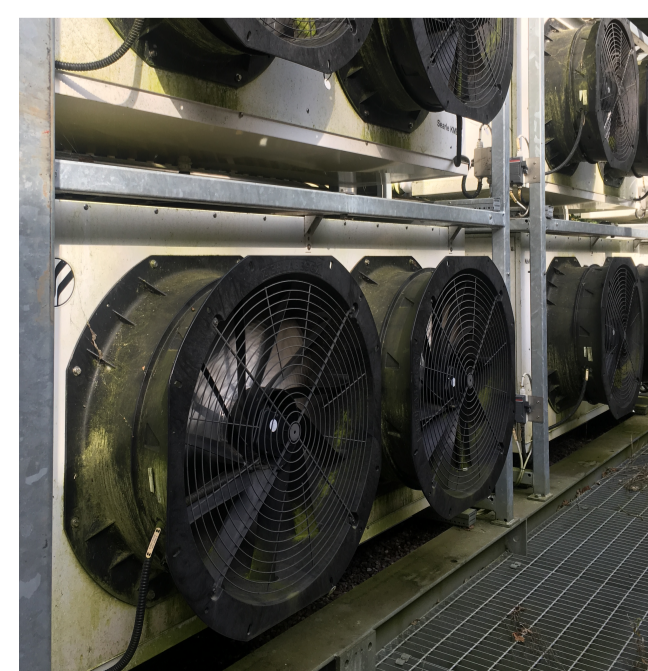
Kelvion Searle evaporator fans and side profile of heat exchanger tubes
