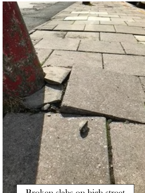
Broken slabs on high street
