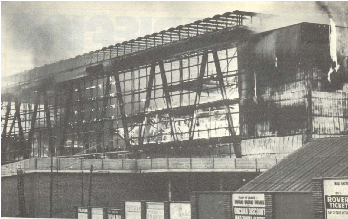
Figure 4.4: The fire starts to burn itself out Only Summerland's V shaped steel skeleton remains (Source: New Civil Engineer , 9th August 1973, page 12)
