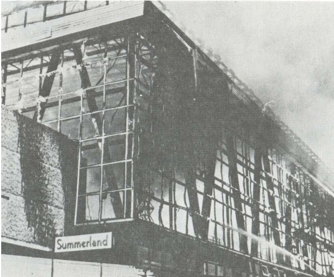
Figure 6.22: Venting of the fire caused by the destruction of the Oroglas promenade wall (Source: Pym, 1977, page 88)
