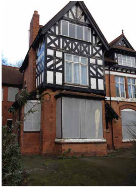
FIGURE 1.2 Homes waiting for refurbishment in Lozells, Birmingham. Source: author
