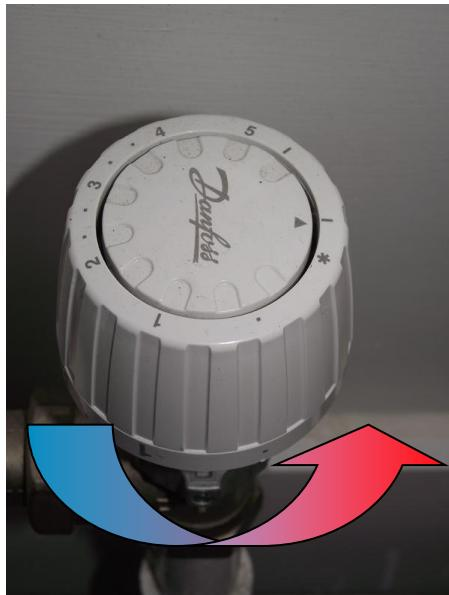
To adjust the heating temperature, turn TRV (adjustable valve on your radiator: **0 = low** and **5 = high**).
