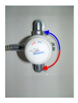
To increase the temperature turn the main body of the shower unit, the further you turn the control the hotter the water temperature. As a guide the control indicates settings from 1-9 if you feel the temperature is too hot or only warm at level 9 then please contact reception and ask to have the temperature checked and adjusted if necessary.
