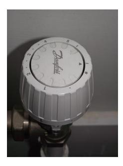
In addition, there is thermostatic radiator valve (TRV) on the radiator in your bedroom and these can be set to your individual requirements. To adjust the heating temperature, turn the TRV on your radiator: 0 = low and 5 = high.
